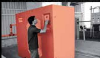
Checking compressor and pipings
