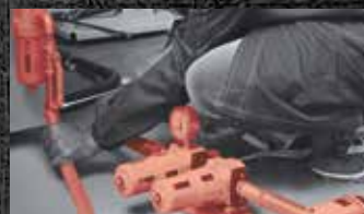
Checking cfm consumption and leakages
